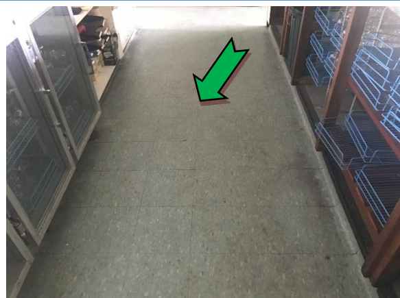
Photo 6. Interior, club house, floor coverings – non asbestos-containing vinyl floor tiles.
