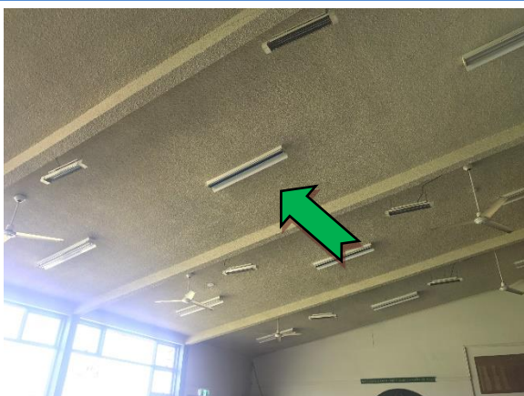
Photo 5. Interior, ground level, club house, ceiling coating – non asbestos-containing vermiculite.
